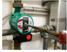
With a large screwdriver unwind the cap.
